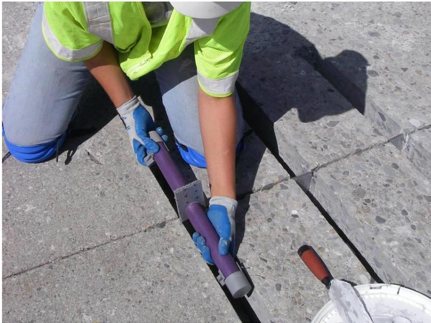
**Figure 8. Inserting dowel bar assembly into slot. (Photo Courtesy of Jeff Uhlmeier, WSDOT)**
