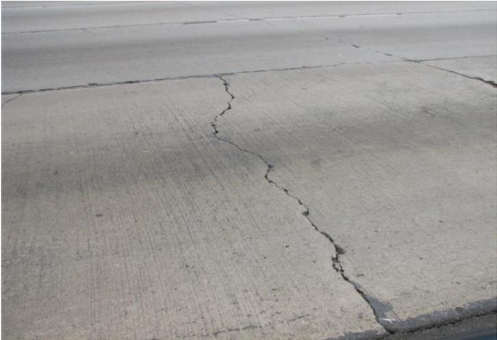
Figure 24. Midpanel cracking on an RSC slab on I-5 in Los Angeles County.
