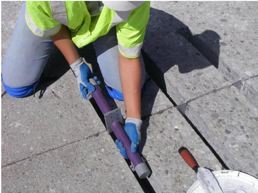
**Figure 8. Inserting dowel bar assembly into slot. (Photo Courtesy of Jeff Uhlmeyer, WSDOT)**
