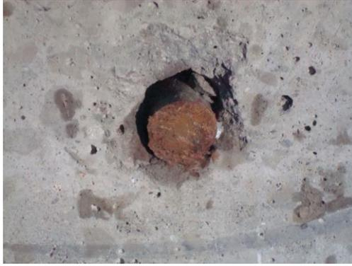
**Figure 17. Poor anchoring of dowel into hole that resulted in faulting of the transverse FDR joint. (Photo Courtesy of Mark Snyder)**
