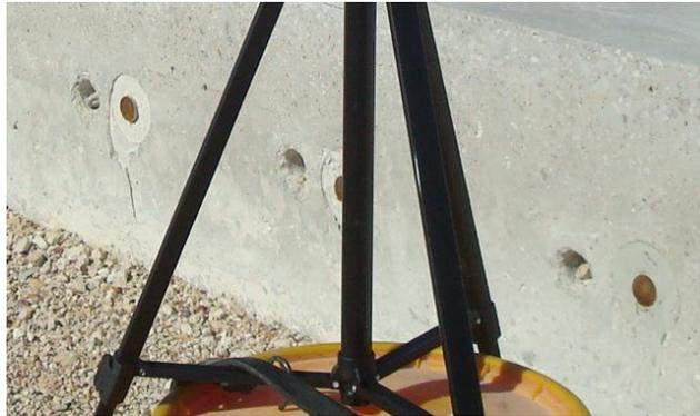
**Figure 18. Use of grout retention disks provides good coverage. (Photo Courtesy of Mark Snyder)**
