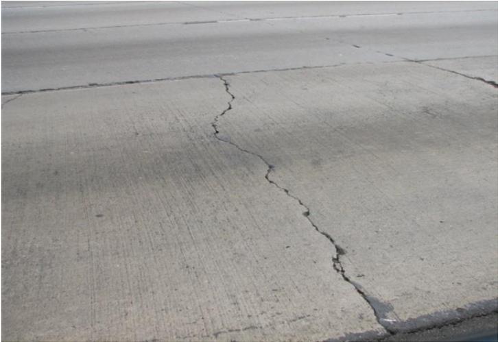
Figure 24. Midpanel cracking on an RSC slab on I-5 in Los Angeles County.
